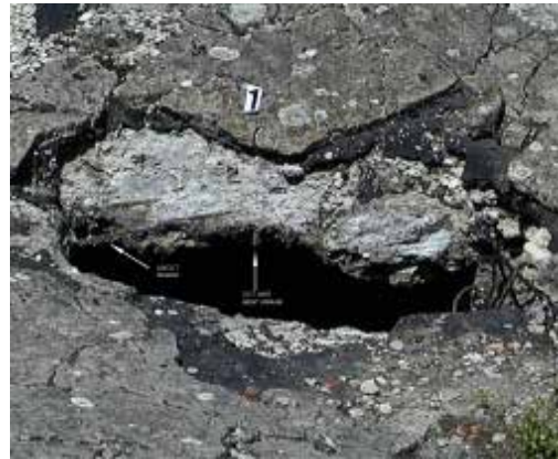
Fig. 2. Zyklon Hole 1, Crematorium II. Tarpaper separating concrete layer below and sand-cement layer above is visible. Source: Daniel Keren et al., “The Ruins of the Gas Chambers: A Forensic Investigation of Crematoriums at Auschwitz I and Auschwitz-Birkenau,” Holocaust and Genocide Studies , vol. 18, no. 1 (Spring 2004): 68–103.
