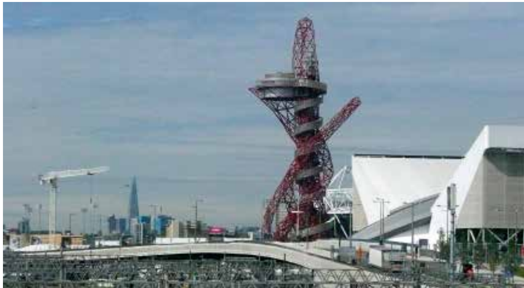
Narrator 2: Rising to the soaring height of 114.5 meters and outstripping even the Statue of Liberty by two meters, the ArcelorMittal Orbit boasts an impressive compendium of statistics: 1,500 tons of steel, 35,000 bolts, 19,000 liters of paint, 770 visitors per hour and 5,000 per day, vistas stretching 20 miles into the distance, and an overall price tag of £22.7 million, £19.6 million of which was funded by ArcelorMittal.
