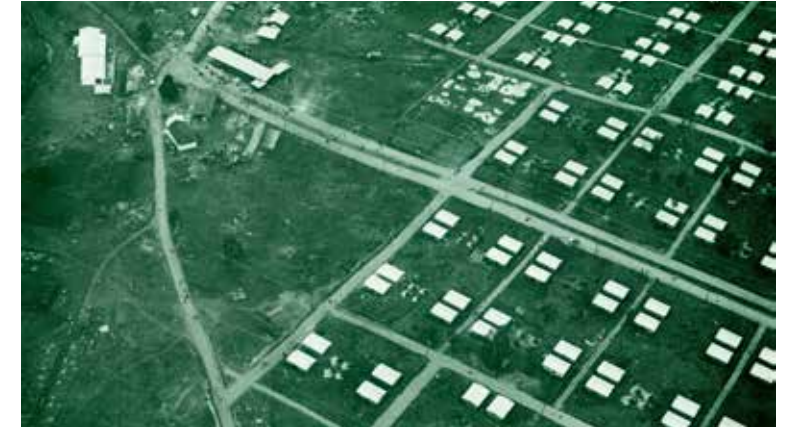
Fig. 21. Aerial view of a part of the newly built model village of Acul. Source: Magazine of the Guatemalan Army, Polos de Desarrollo y Servicios (1984).
